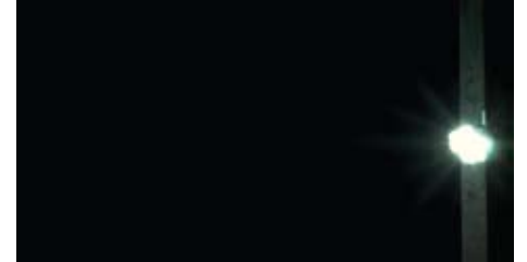
Arc fault delivered to a circuit protected by Amp-Trap 2000 fuses
