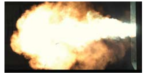
Arc fault delivered to a circuit without fusing
